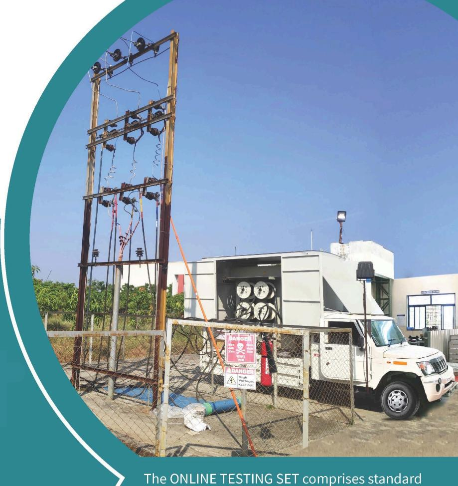
HT TVM, CTs, PTs and switching device. The OLTS is competent to test the entire Metering Set comprising of CTPT unit, TVM and Control cable in on-load condition without interrupting the Power supply.
