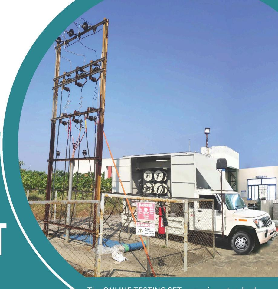
The ONLINE TESTING SET comprises standard HT TVM, CTs, PTs and switching device. The OLTS is competent to test the entire Metering Set comprising of CTPT unit, TVM and Control cable in on-load condition without interrupting the Power supply.
